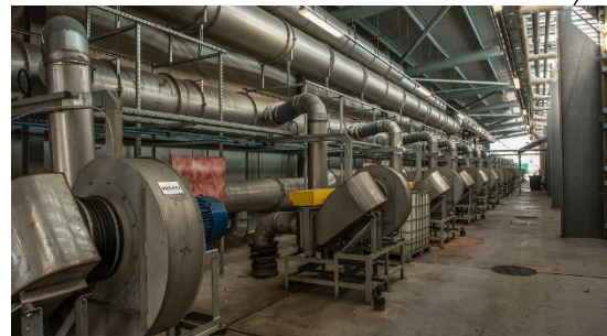
(2) VENTILATION SYSTEM FOR EXHAUST AIR EXTRACTION
