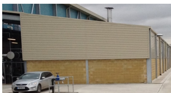
(3) BIOFILTER FOR THE PROCESS ODOURS ABATEMENT
